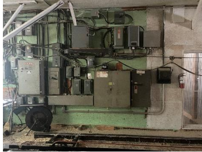
Electric breaker box with soft start
